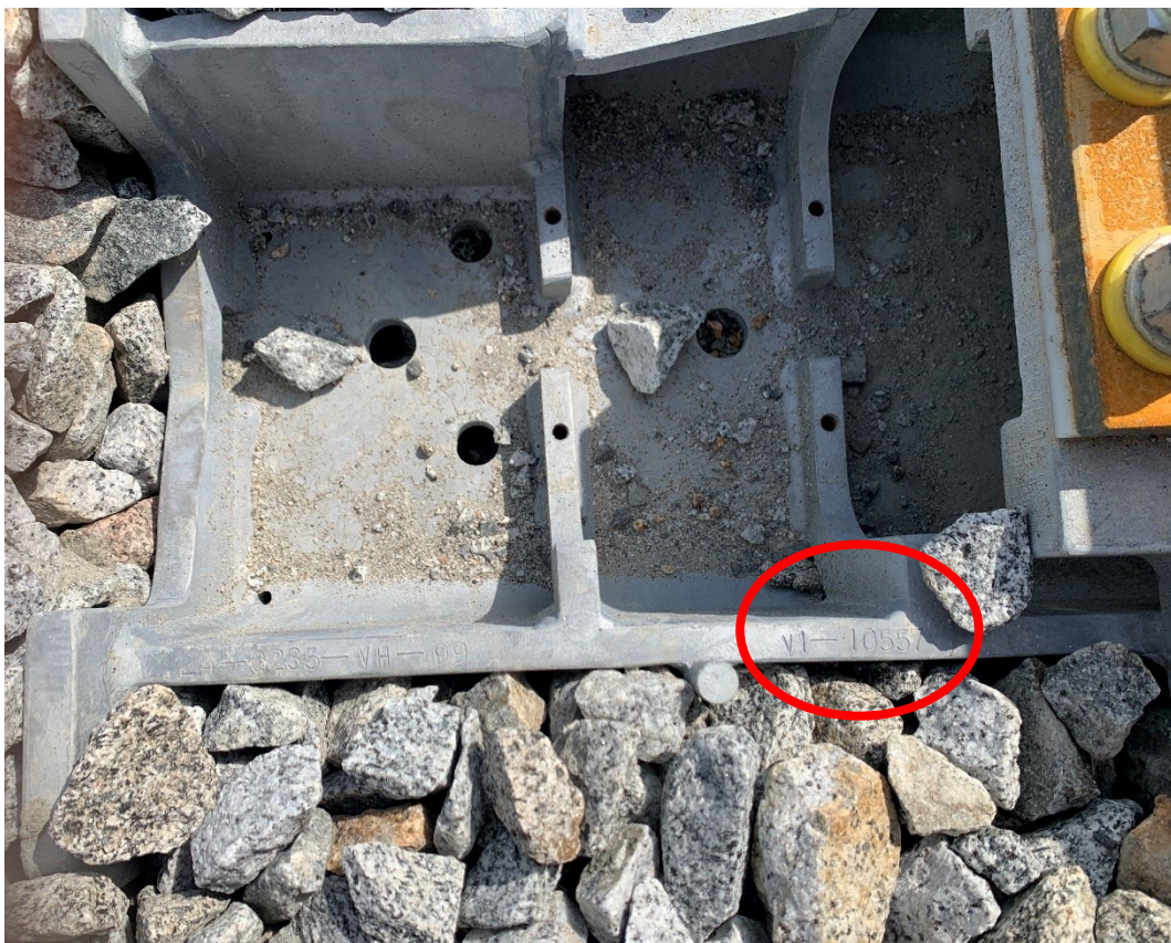
Fig. 20 Identification of a narrow trough sleeper
