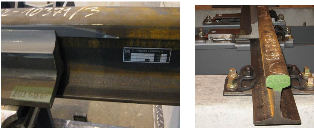
Figure 13 – Example of switch identification: side view and front view
