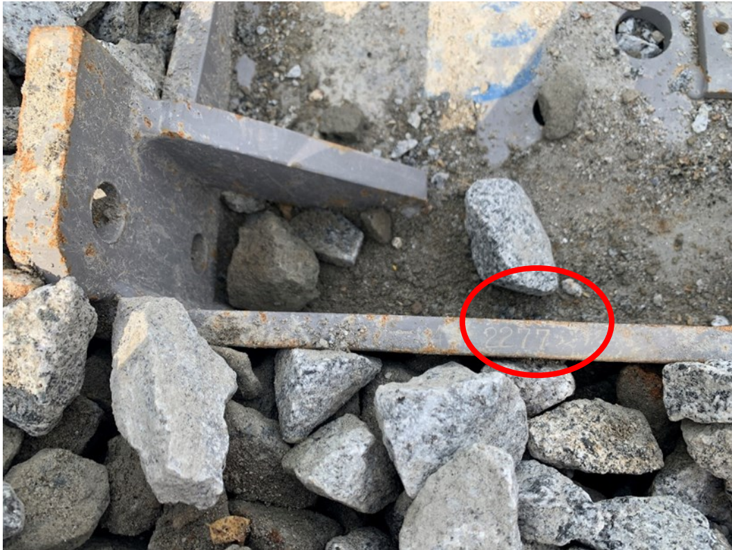
Fig. 19 Identification of a wide trough sleeper
