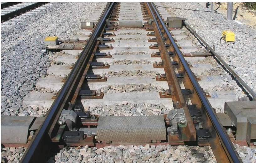
Figure 1 – Switch of a simple turnout
