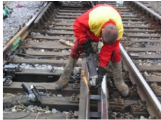
Figure 54 – Manual grinding with an abrasive disc
