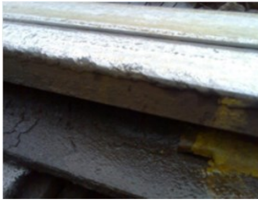
Figure 55 – Switch rail lap
